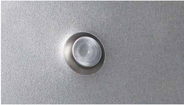
RESULT OF THE INSTALLATION OF SELF-PIERCING RIVET
